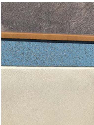
04 A contrasting polished band between the upper edge and pool interior.
