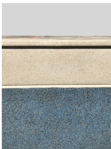
08 Traditional coping over a smooth waterline band and exposed aggregate below.
